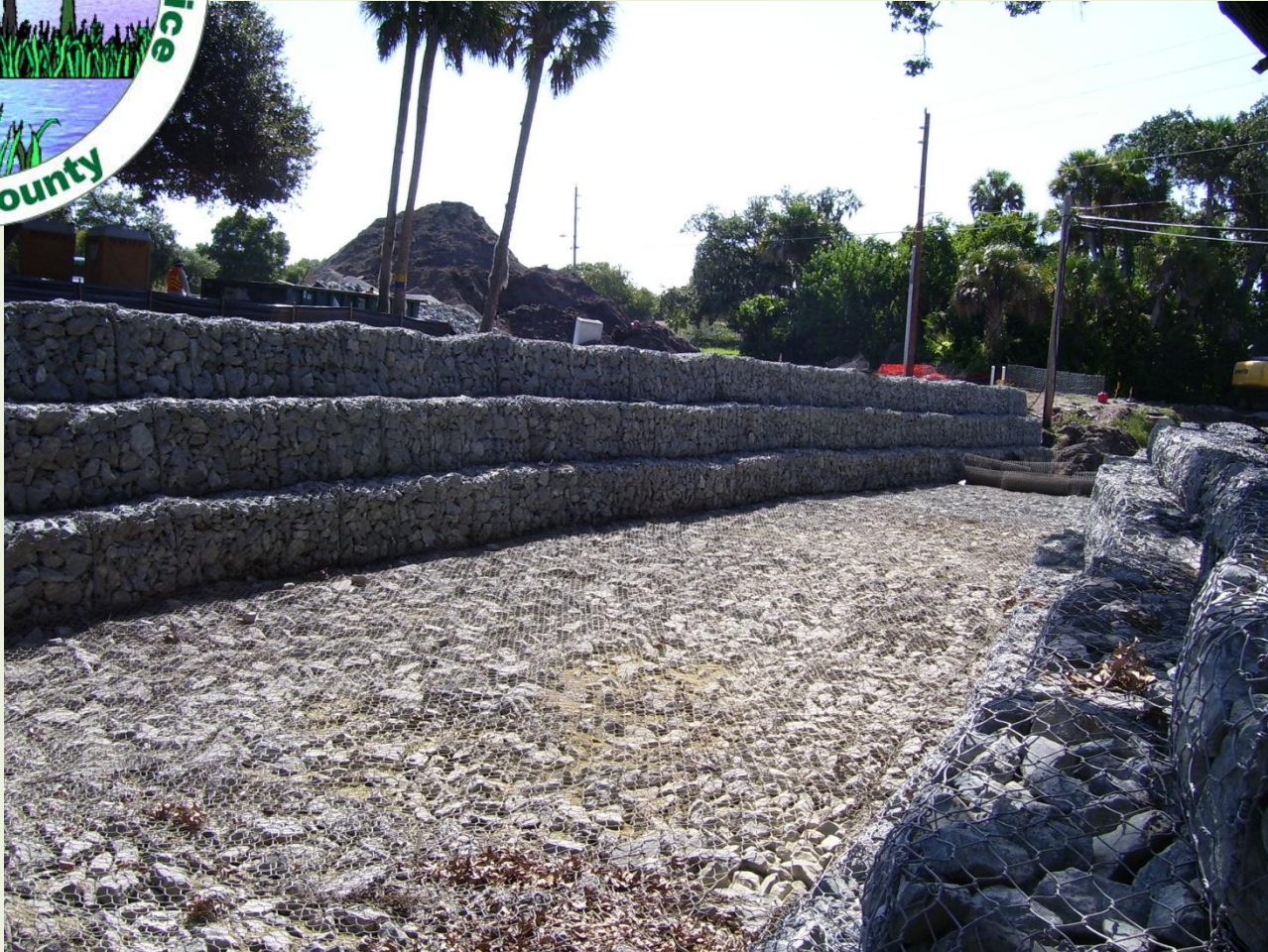
Picture of the M-1 canal construction progress August, 2010
