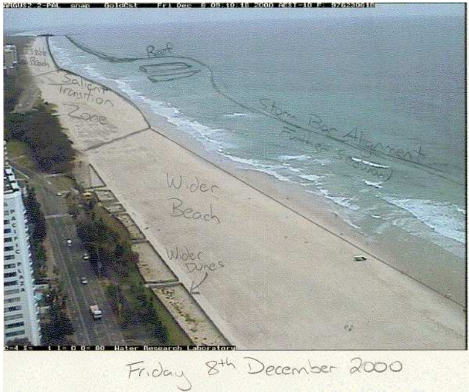
Figure 1 - Annotated Photo of Narrowneck Salient
