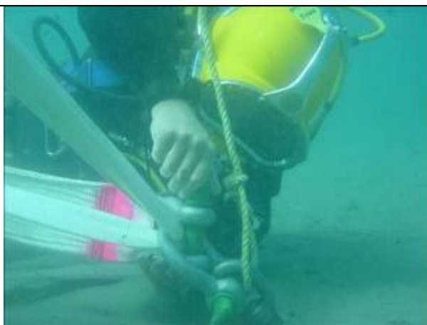
Reef Section Securing to Seabed
