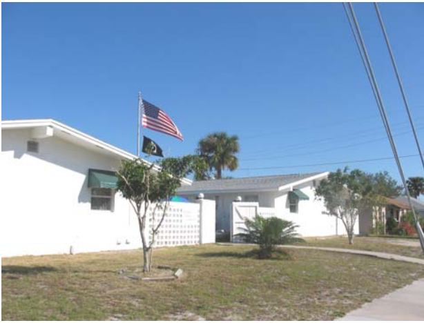
Front Entrance to Veterans Center
