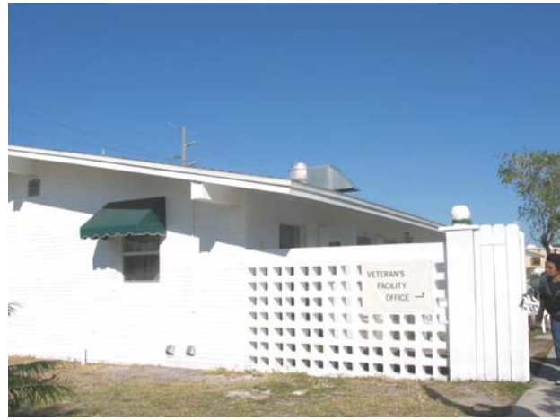
Front Entrance to Veterans Center
